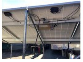
Daylight Inverter with power receptacle
