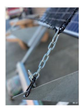
5. Install a single carabineer (D) on the triangle supports going halfway around the net and attach the net to the supports. The other half of the net will use a chain tensioner (C) (2 carabineers and an 18" chain) to secure the net to the supports. When installing the chain tensioners, pull the net tight and clip the carbineer into the chain link that will keep the net the tight.
